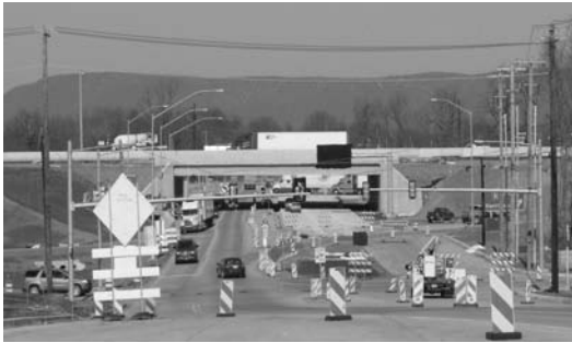
PA 465 – South of Interchange
