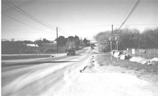
PA 465 – South of Interchange
