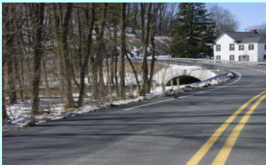
Roth Road Bridge
