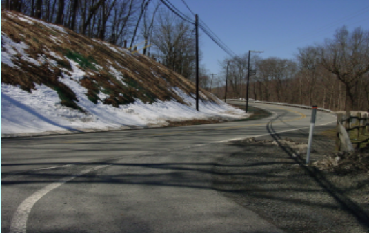
Roth Road Bridge
