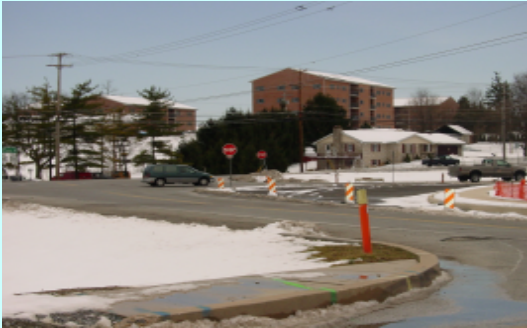
PA 116 Spring Grove Roundabout
